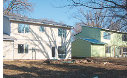
Superefficient houses don't have to look strange. These two houses, part of the Passive House Conference's home tour, use about 10% of the heating energy required by normal houses.
